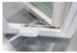
Pictured above new modern lock and handle paired with stainless-steel operator, hinge track, and hinge arm
